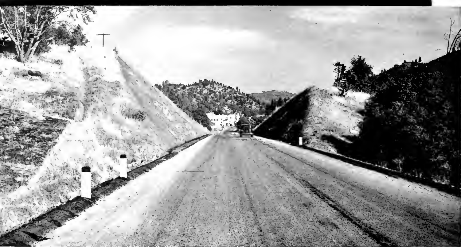
Road mix on gravel base surfaces a relocated section of State Route 18 in a mountainous area
